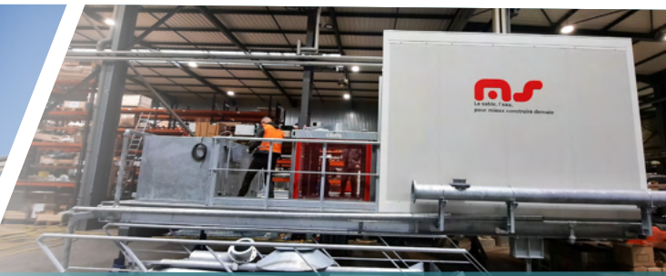
02 Pre-wiring in the workshop
